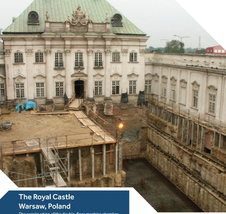
The construction of the double-floor machine chamber 10m below the courtyard of the 18th-century palace was highly restricted by the presence of historic structures in the subsoil, giving the excavation pit a complex layout. The design and build of the excavation support system was done by Keller Polska and was successful in protecting adjacent buildings. Lateral displacement of the palace wall not exceeding 4mm.
